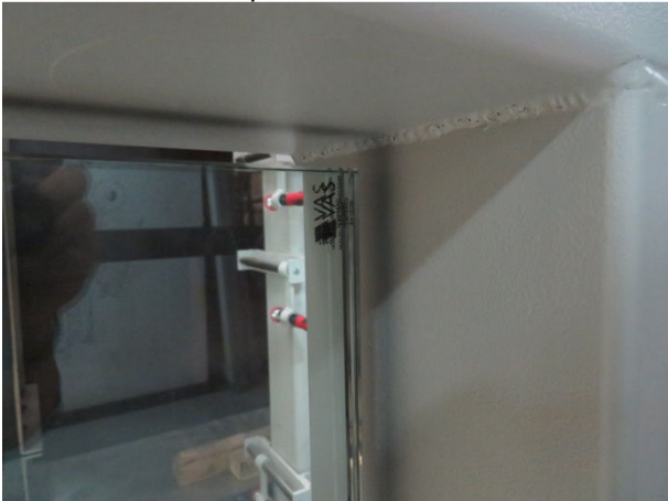
Picture 3 Corner of glazing at top
