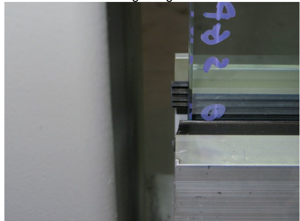
Picture 6 Glazing in Aluminium profile
