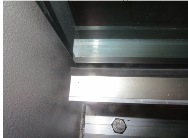
Picture 4 Corner of glazing at bottom
