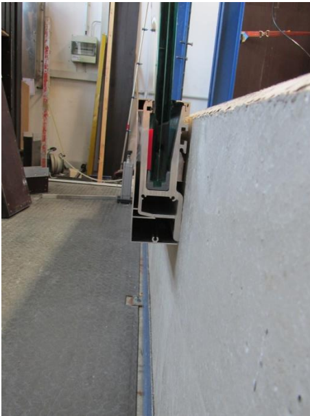
Picture 3 Static outward test - Test with 1.0 kN/m
