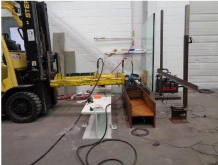
Photo No. 1 In-Fill Load Test at Bottom of Infill
